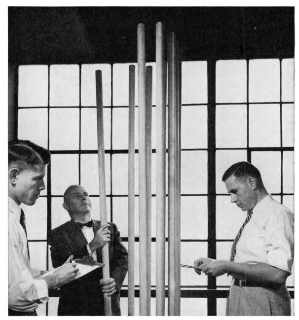
**Electric company engineers** arrange full-size wooden models of the uranium rods that are the atomic fuel for certain types of atomic-electric plant. Several dozen such rods of uranium can supply enough heat to generate a whole year's electricity for a good-sized city.
